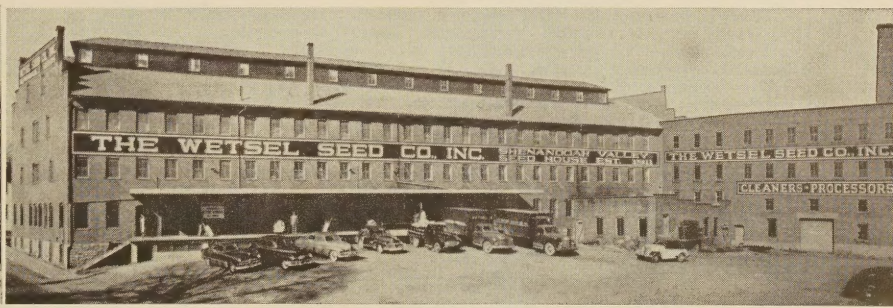
Gay Street Warehouse, devoted to the storage of seeds and other merchandise and cleaning of grains and grass seeds.
